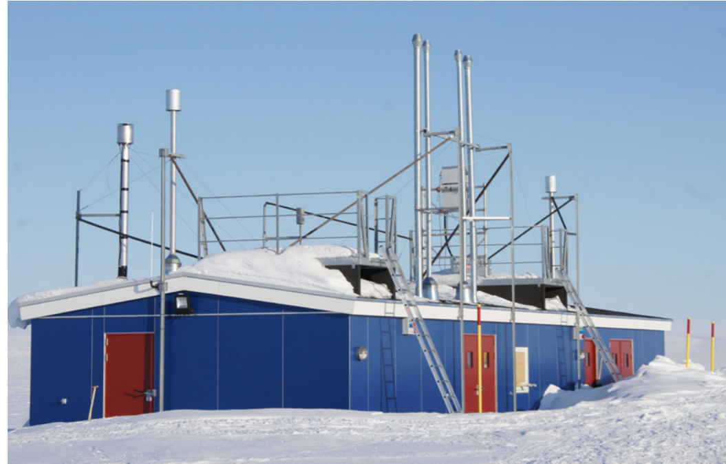
Figure 4. The air measurement facility is equipped with specially designed inlets for a range of different air measurements.
